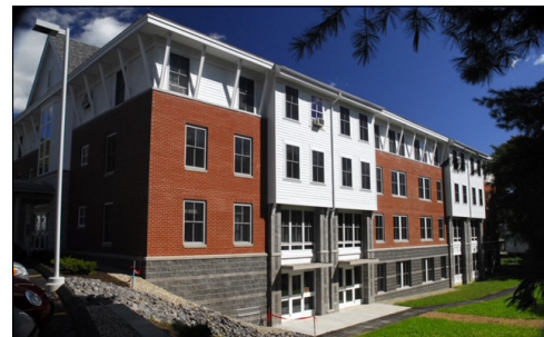
Golder Commons 6 Lincoln Street • 26 Family Apartments
