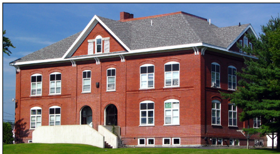
School House Commons 87 Bridge Street • 8 Family Apartments
